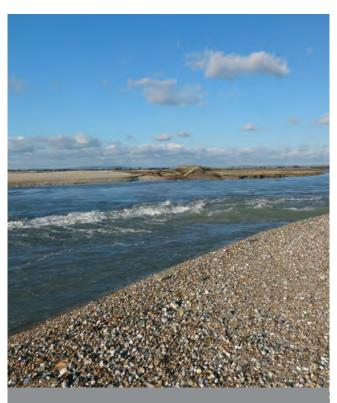
Figure 2.4: View of the breach made in the existing shingle bank at Medmerry managed realignment site. Medmerry, on the south east coast of England, is the largest managed realignment on the open coast in the UK and Ireland. The shingle bank defence was breached in 2013. Photo: Mark Schuerch.
