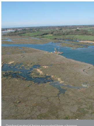
Dredged material being excavated from a hopper barge and hydraulically pumped via pipeline, in order to recharge an eroding marsh. Photo: Suave Air Photos, taken March 2012
