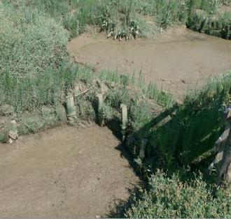
Figure 5.7: Installation of one of the coir roll structures in November 2018 (left) and example coir structure in summer 2019, by when plants had begun to grow (right). Photo: Essex Wildlife Trust.
