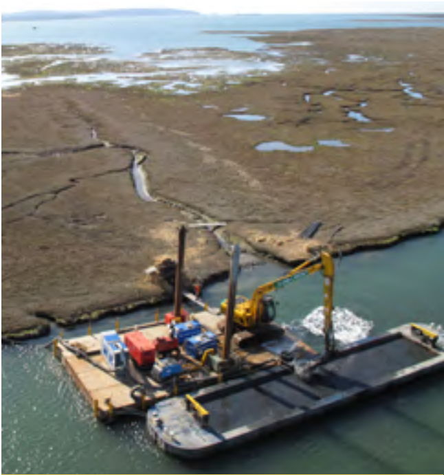
Dredged material being excavated from a hopper barge and hydraulically pumped to restore an eroding marsh (Land and Water Ltd.).
