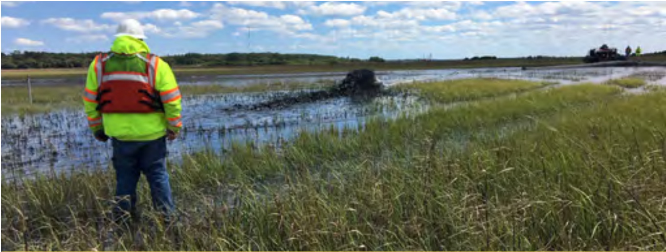
Monitoring dredged sediment placement as part of a 2 ha thin layer placement project at Jekyll Creek, USA (Clay McCoy, USACE Jacksonville District).
