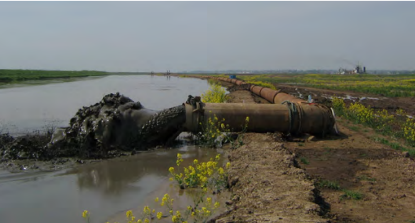
Figure 2.9: Hydraulic disposal by pipeline and the last disposal of 550,000m³ of fine sediment prior to breaching of the flood defences at Allfleet’s Marsh, Crouch Estuary, Essex (ABPmer).
