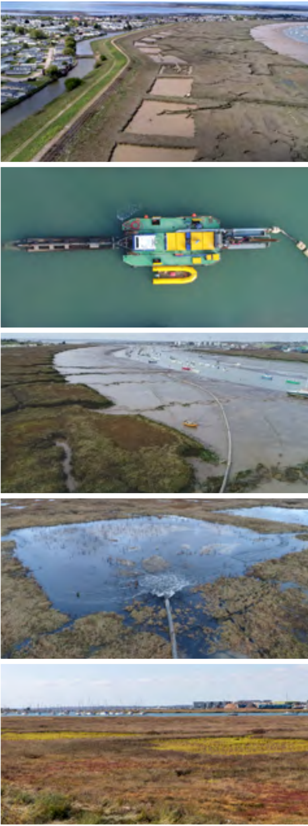
Figure 2.8: St Osyth borrow pits, Colne Estuary, Essex, from top: borrow pits prior to disposal; cutter suction dredger in operation; pipeline used for transport and disposal; fine sediments being disposed by hydraulically pumping via pipeline; and subsequent colonisation of the borrow pits following disposal (Exo Environmental Ltd.).
