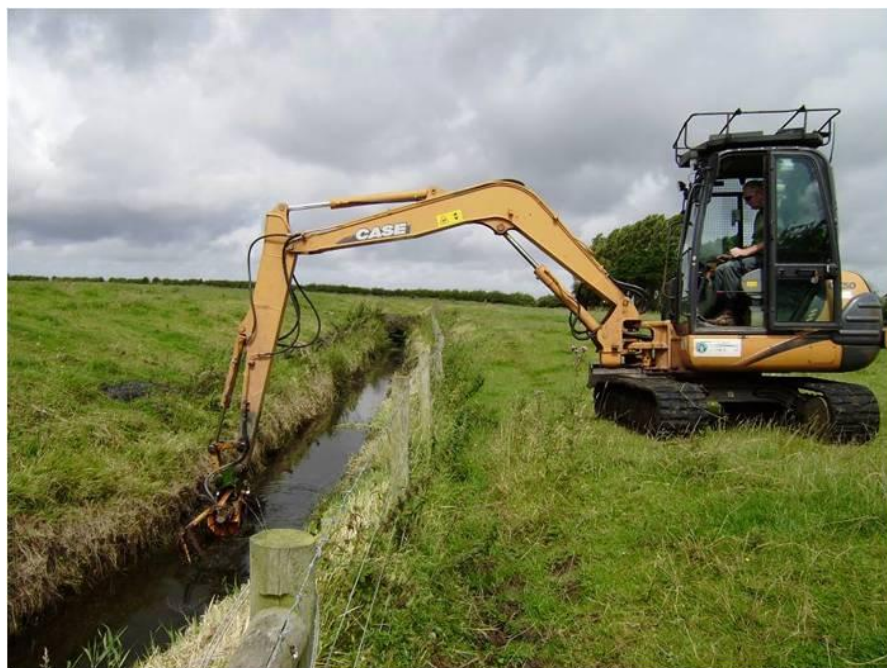
Figure 4: Use an appropriate sized machine and bucket
