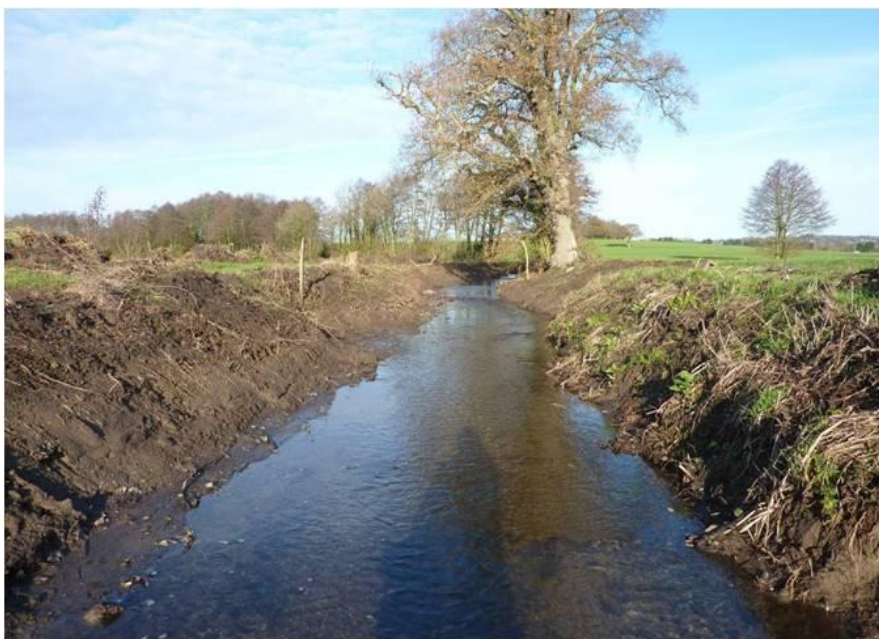
Figure 6: You should not leave banks bare or exposed after de-silting
